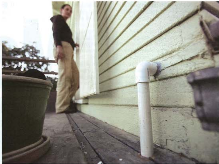
Laura Allen (facing page), cofounder of Greywater Action, installed a drip-irrigation system at a client's home in Oakland, Calif. A three-way valve (left) diverts gray water from the washing machine (above, left) to new bamboo plants outside. A pipe from the laundry (above, right) carries the gray water outside. Users must be particular about detergents so as not to damage plants.
